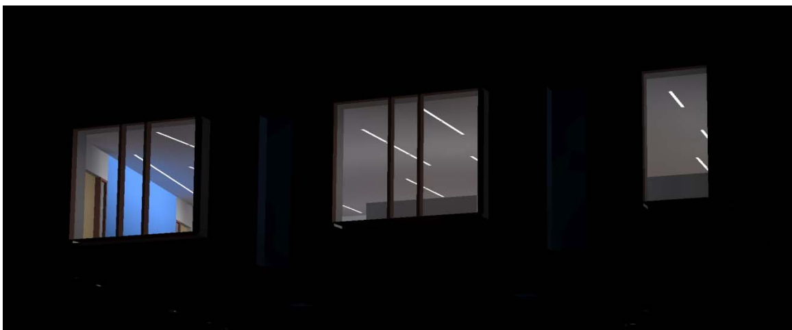
Exterior View from North
